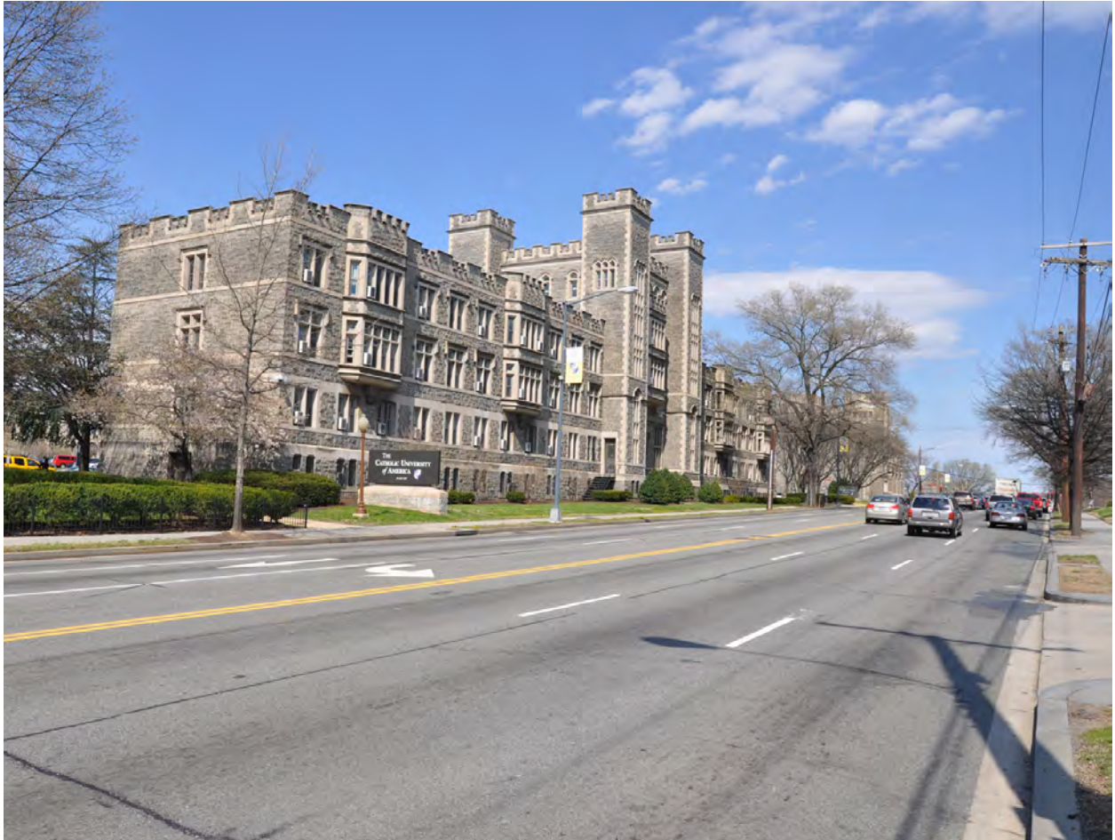
Michigan Avenue Existing Condition
